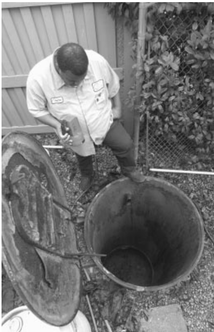
Photo by John Covington/Savannah Morning News A wastewater vacuum truck operator inspects a trap which has collected grease from Savannah's sewer system.
